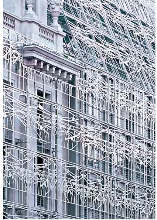
This veil of ornamental, laser-cut 12 mm stainless steel panels overlays the different parts of the Ministry of Culture building in Paris.
