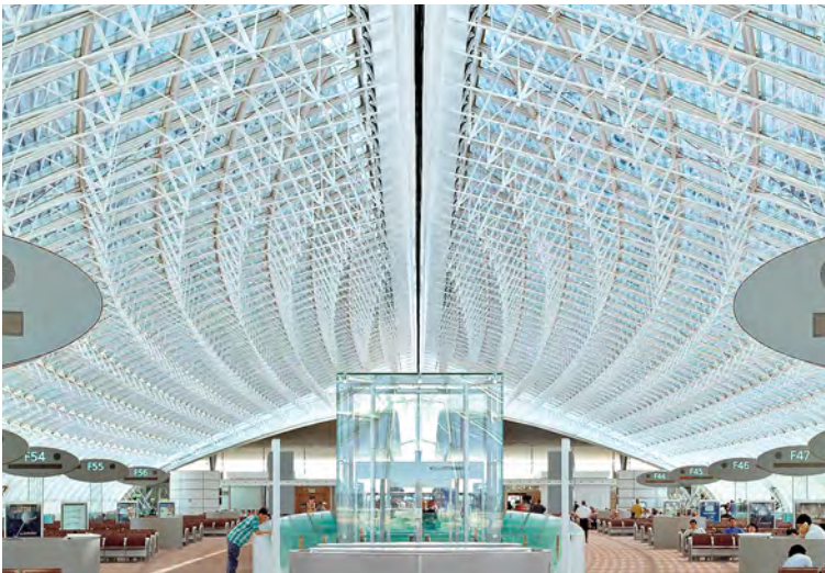
In Charles-de-Gaulle Airport in Paris, trapezoidal stainless steel sheet with 68 mm perforations is mounted on the outside of the glazed departures hall to protect the interior against the sun.
