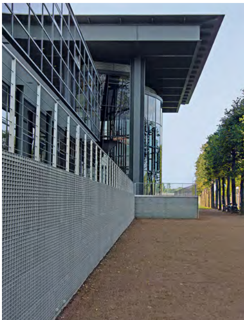
Welded stainless steel grating is used as solar shading on the Mediathèque in the French town of Sélestat.
