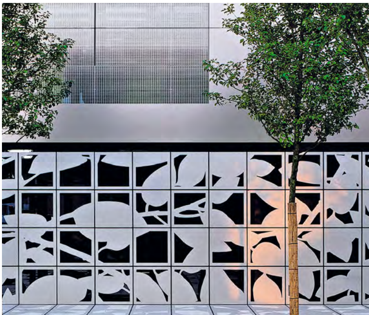
Floral designs, laser-cut out of 5 mm stainless steel panels, cover the 3 m high ground floor of this administration building in Reutlingen.
