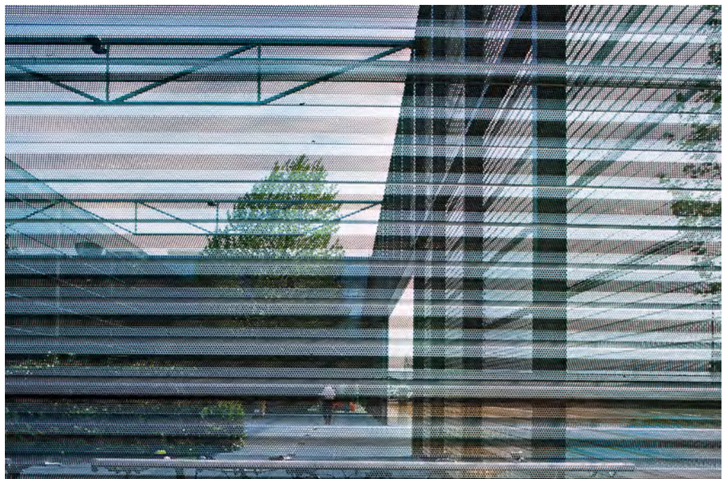
In Charles-de-Gaulle Airport in Paris, trapezoidal stainless steel sheet with 68 mm perforations is mounted on the outside of the glazed departures hall to protect the interior against the sun.
