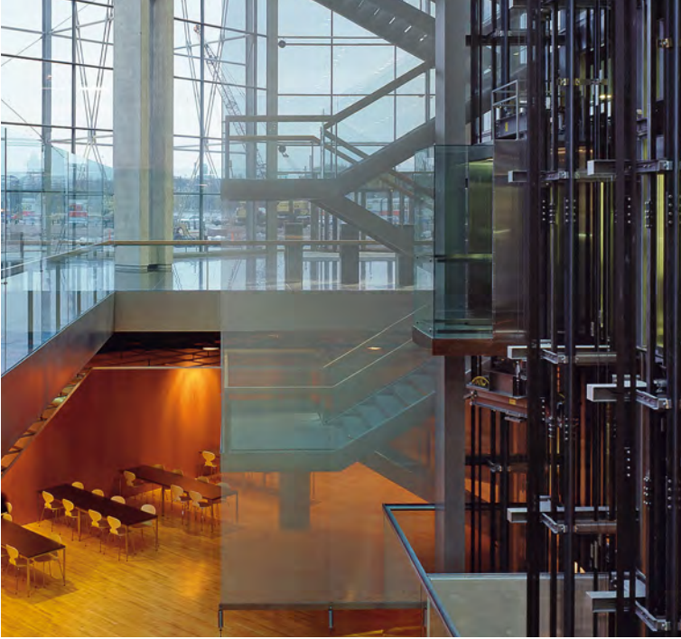
A woven panel stretching up nine storeys forms the parapet of the staircase in the atrium of the Sanoma building in Helsinki.
