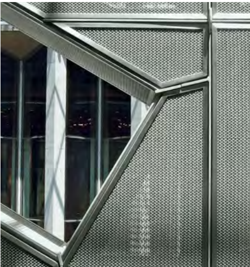
The extensive wall cladding in the National Gallery of Victoria, Melbourne, is made of woven stainless steel fixed in a perimeter frame.
