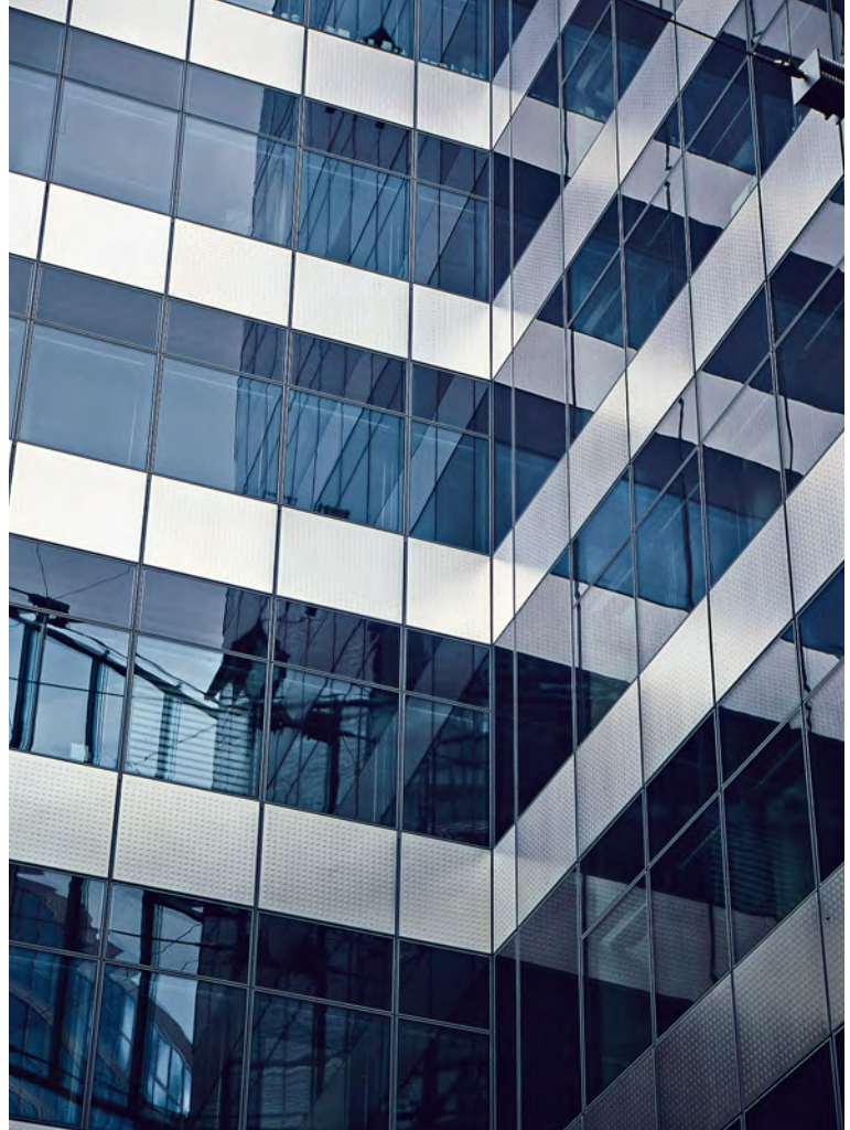
Juxtaposed against the glass, the high surface flatness of the embossed panels becomes evident.
